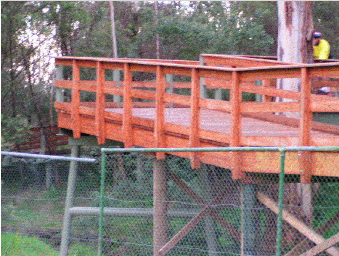
Proximity of Home Run Fence to footbridge (note top rail of fence parting way)
