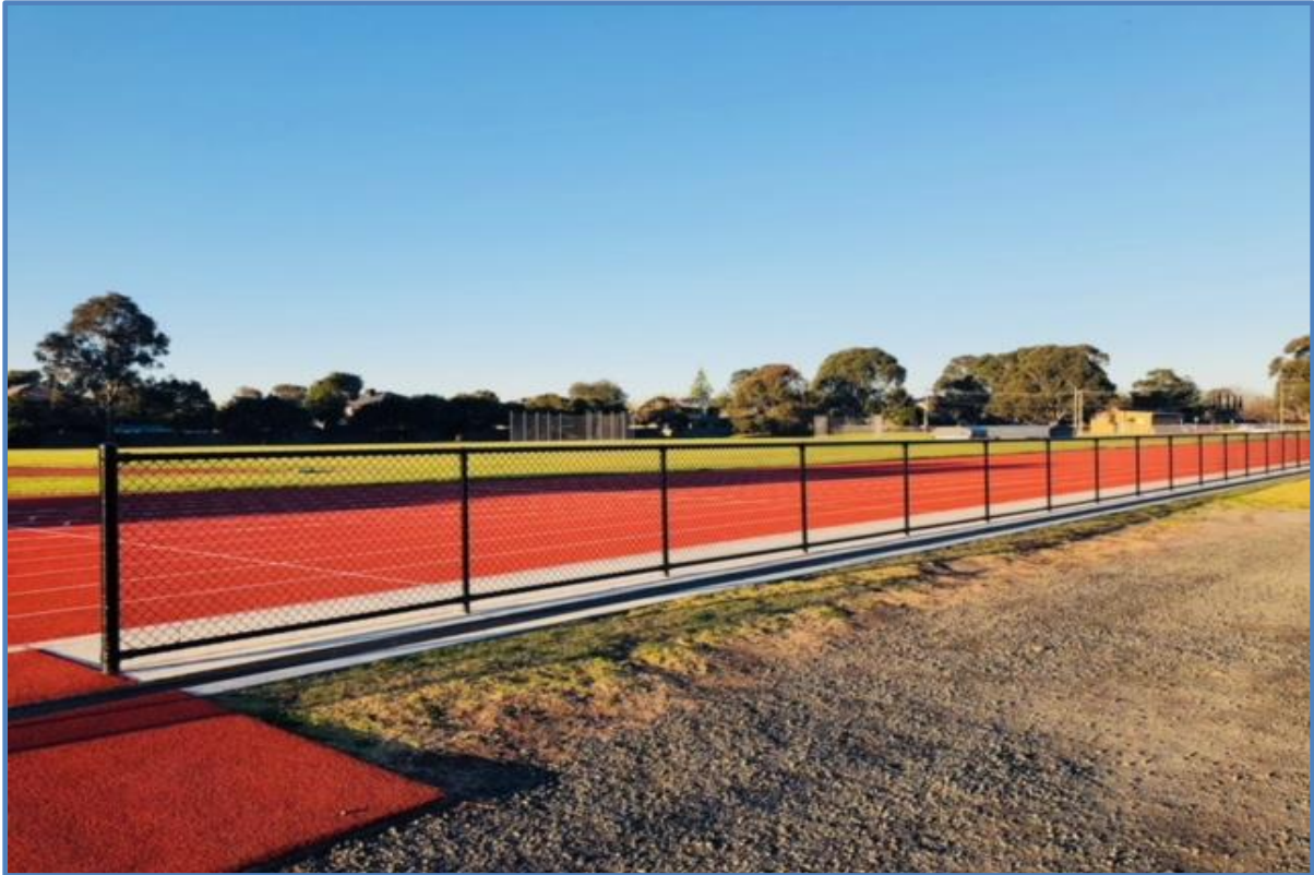
Athletics track perimeter fence (facing outwards)
