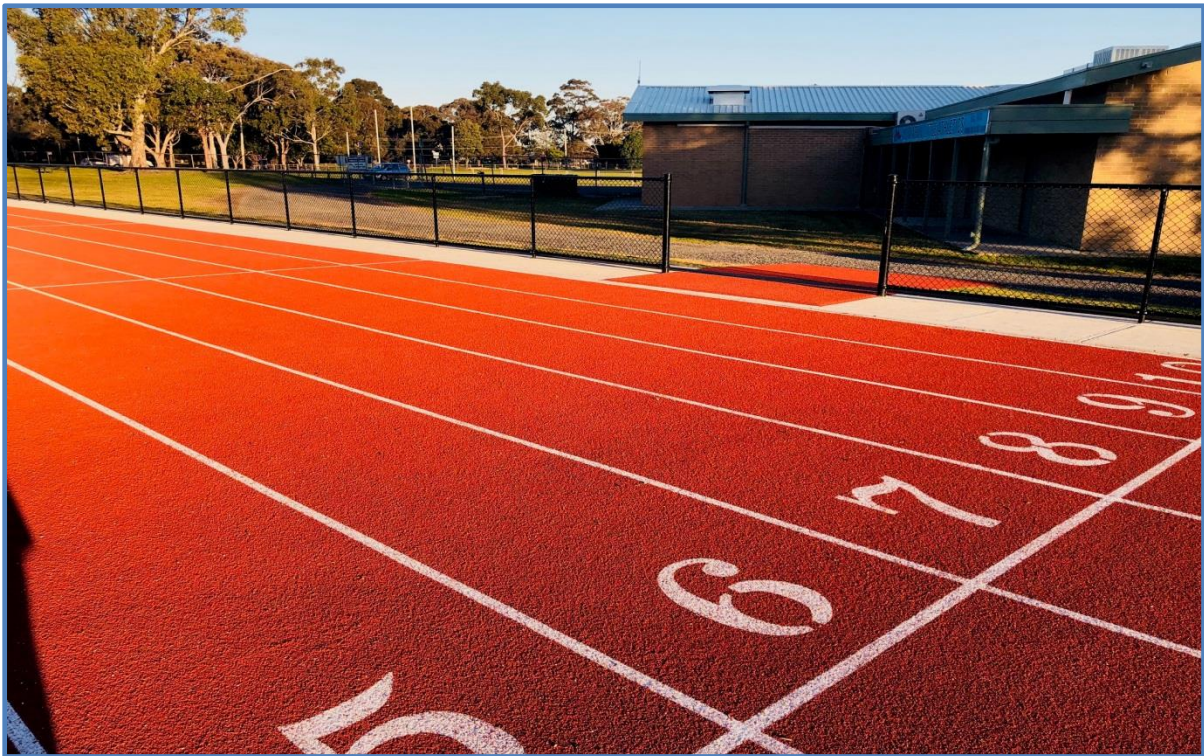
Athletics track perimeter fence (facing inwards)
