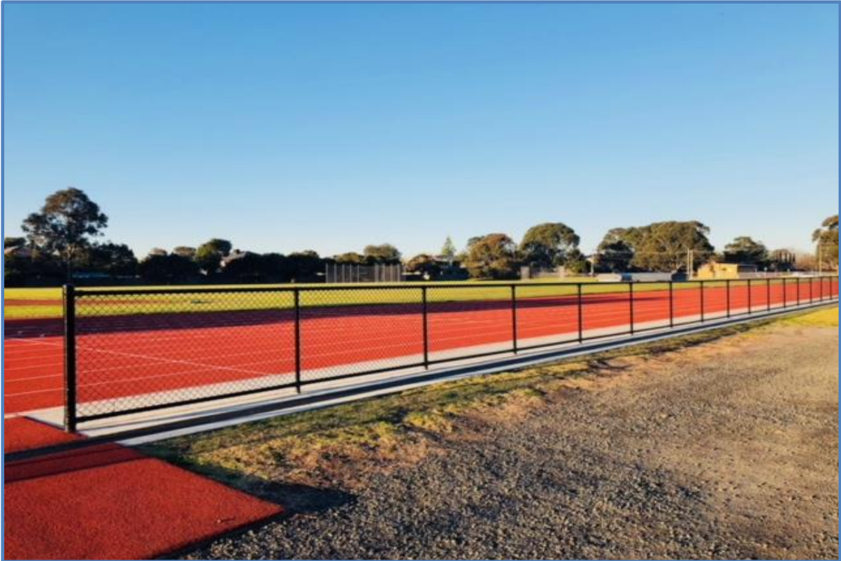
Athletics track perimeter fence (facing outwards)
